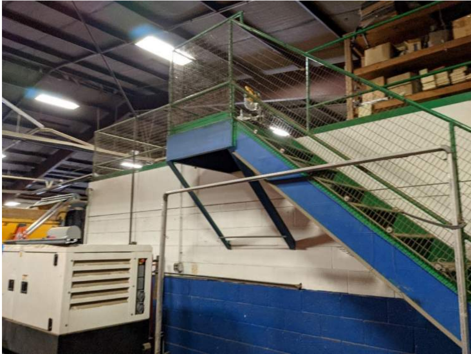
Facing south in southeast portion of garage.
