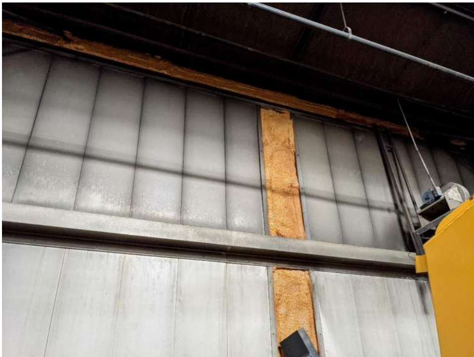
Yellow spray foam at former window openings.
