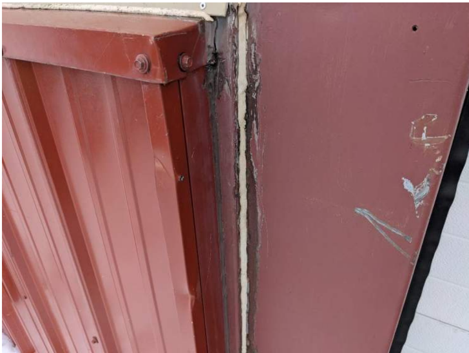
Seam caulk at exterior.
