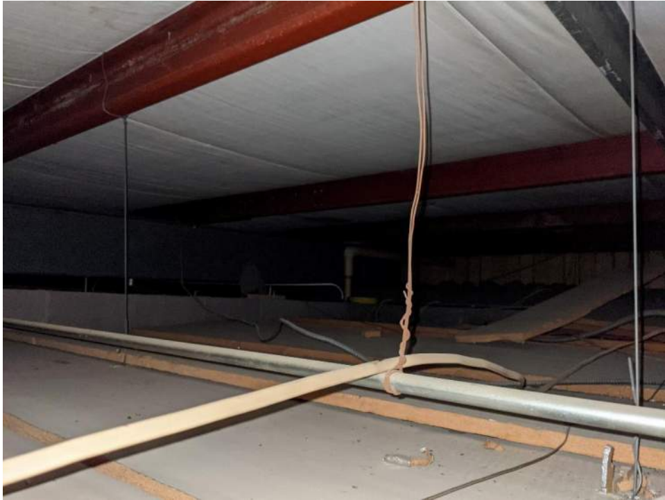
Silver and Loose Insulation Panels above Office
