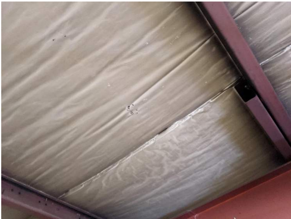
Ceiling insulation and red structural paint.
