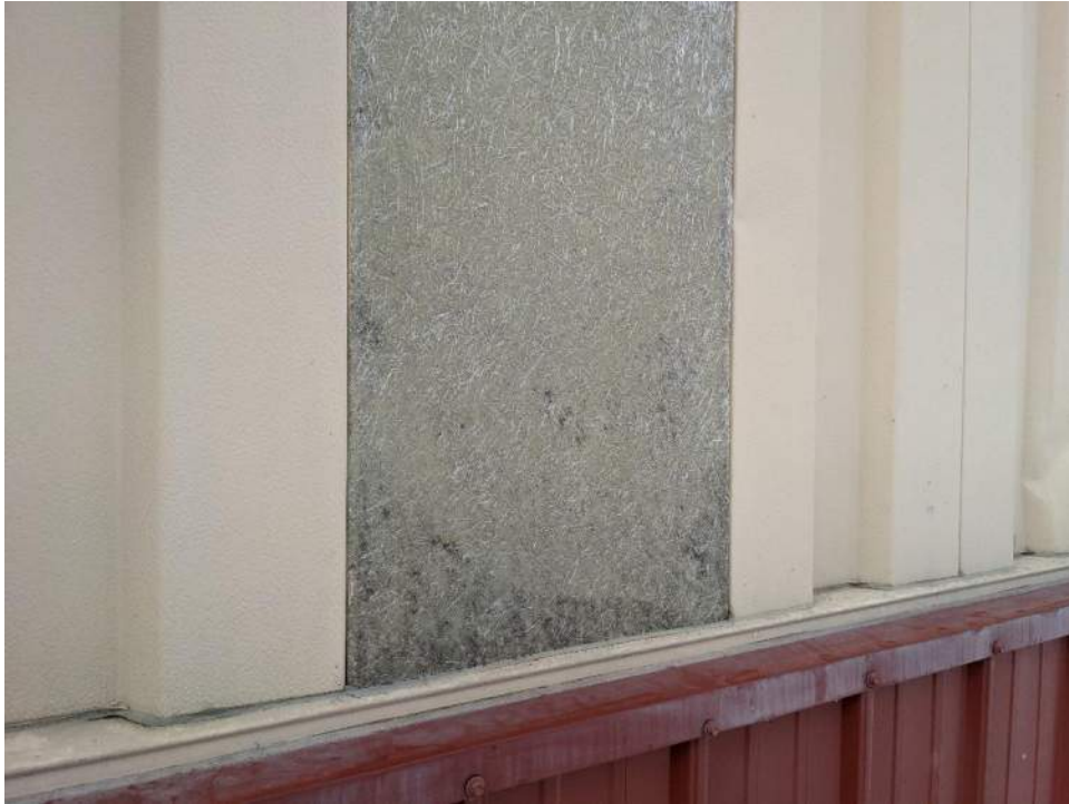
Fibrous board at exterior.
