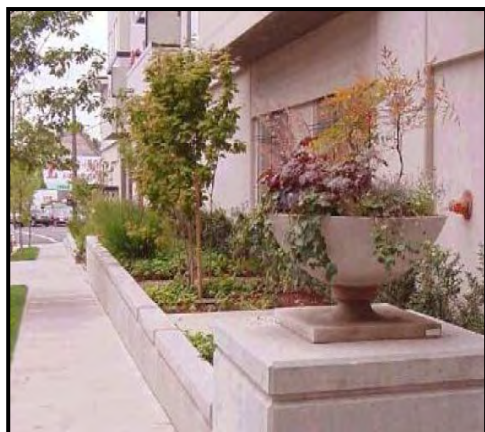
Figure 43: Stormwater Planters (Source: MA EOE, 2005)
