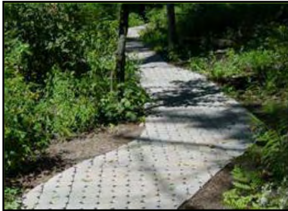
Figure 16: Sidewalk with a permeable paver surface (Source: MA EOE, 2005)
