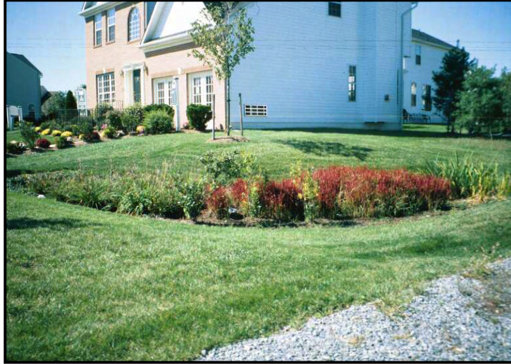
Figure 37: Example of an On-Lot Rain Garden Source (MA EOE, 2005)
