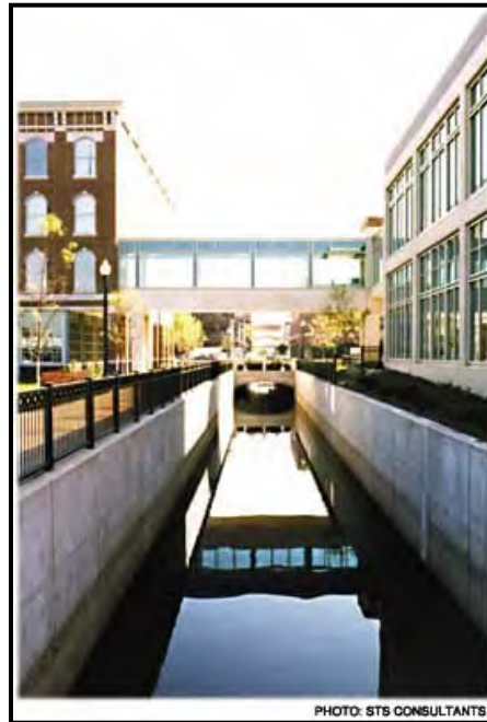
Figure 46: Daylighting Arcadia Creek in an Urban Area in Kalamazoo, MI (Source: Stormwater Magazine, Nov/Dec 2001)
