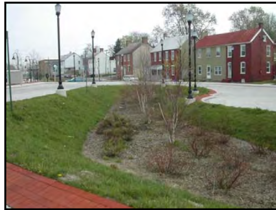
Figure 36: Example of a Bioretention Facility Along Roadway
